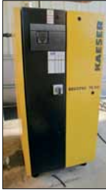
KAESER COMPRESSED AIR DRYER # TE142
